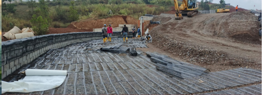
Proses pemasangan Multiblock Retaining Wall
